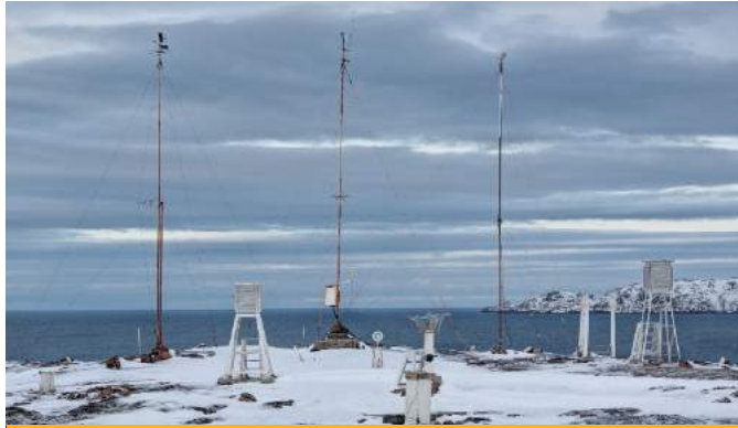
Remote monitoring and communication
