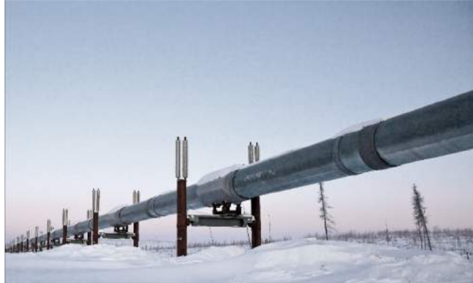
Surveillance and control systems
